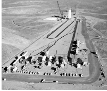
Figure 4. Tower and Cables before Lowering the Rack
