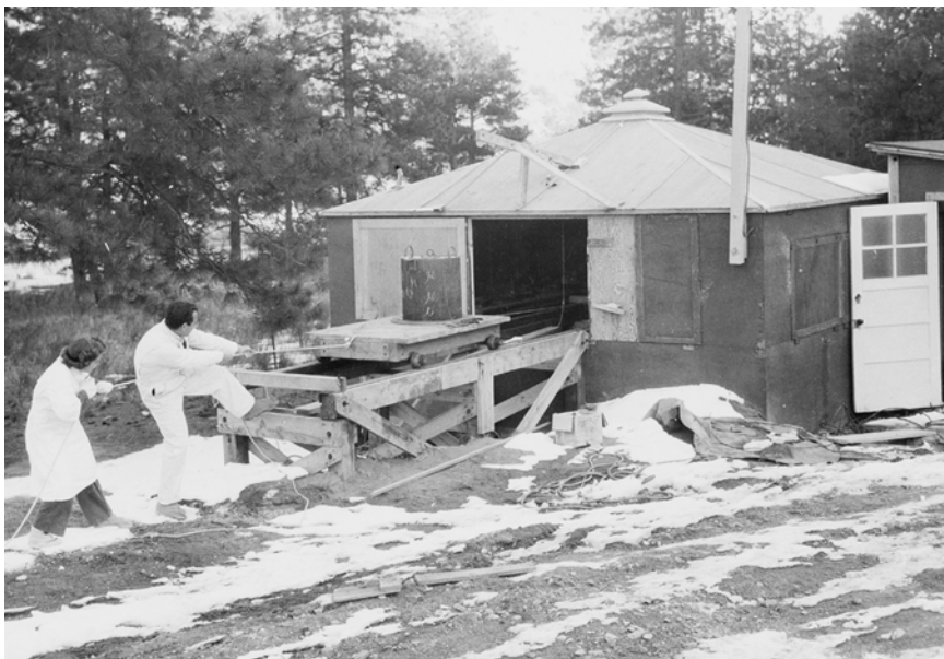
Figure 3. The Radiolanthanum Experiments This photo taken at Los Alamos during the Manhattan Project shows the “remote handling” of a kilocurie source of radiolanthanum located inside a lead container. This strong gamma-ray source would be placed at the center of a hydrotest assembly to measure the areal density of the pit (from the center outward) as a function of time.
